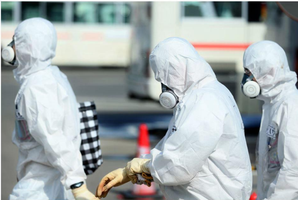
Reactor decommissioning workers wearing protective suits are seen at the Fukushima No. 1 nuclear plant on Feb. 23, 2016. (Mainichi)
