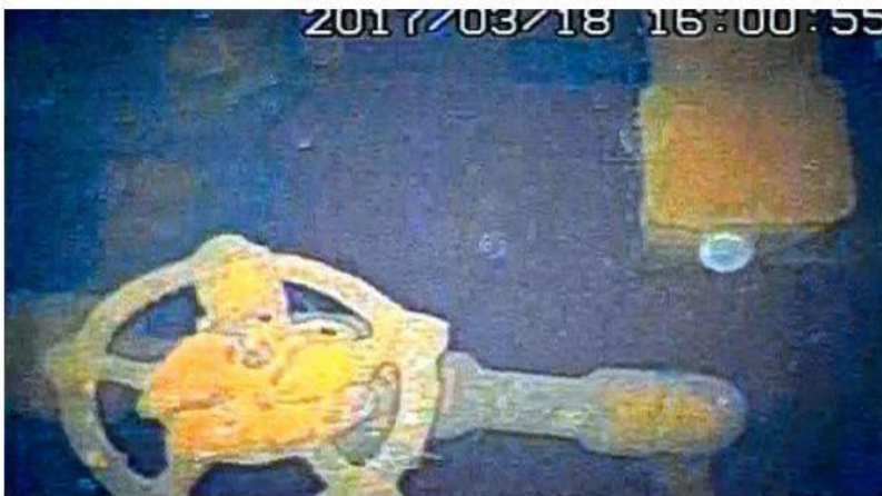
A robot on March 18 took this image of a valve and a pipe in cooling water at the bottom of the containment vessel of the No. 1 reactor at the Fukushima No. 1 nuclear power plant. (Provided by the International Research Institute for Nuclear Decommissioning)
