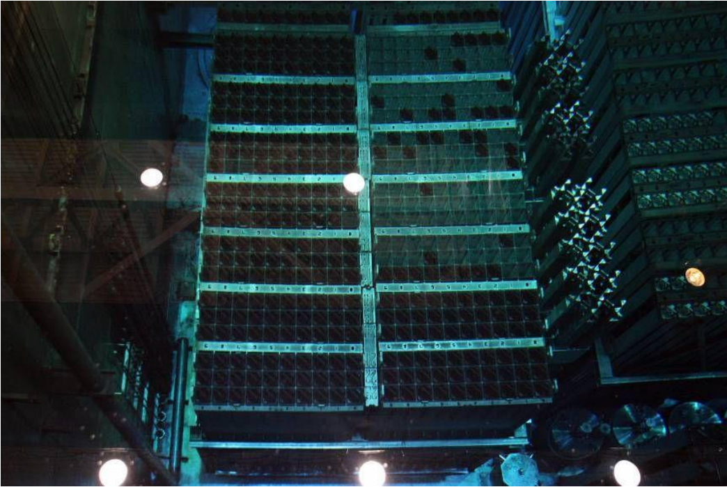
Channel boxes containing fuel rods with plutonium-uranium mixed oxide (MOX) lie in a pool in the building housing the No. 3 reactor at Tokyo Electric Power Co.'s Fukushima No. 1 nuclear power station in the town of Okuma in August 2010. | BLOOMBERG
