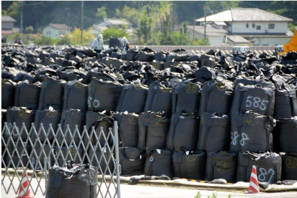
Piles of black bags containing radioactive soil are seen at a temporary storage site in Minamisoma, Fukushima Prefecture, on June 11, 2016. The Environment Ministry is set to conduct a demonstration experiment there possibly later this year, in which radiation doses will be measured on mounds using soil generated from decontamination work. (Mainichi)
