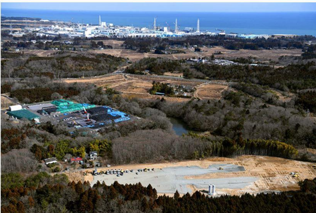
An intermediate storage facility under construction in Okuma, Fukushima Prefecture, in February, with the Fukushima No. 1 nuclear plant in the background (Asahi Shimbun file photo)
