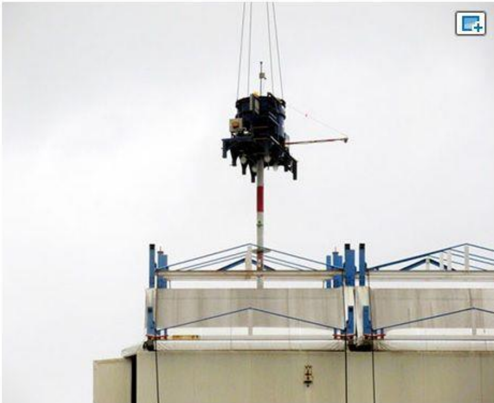
Workers drill into a panel of a canopy covering the damaged No. 1 reactor building at the Fukushima No. 1 nuclear power plant on Oct. 22. (Provided by Tokyo Electric Power Co.)
