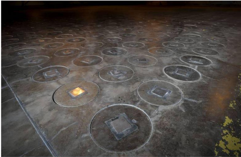
This 2013 file photo shows radioactive waste sealed in large stainless steel canisters under a five-foot of concrete in a controversial storage facility near Aiken, South Carolina. The Ministry of Economy, Trade and Industry has plans to dispose of Japan's nuclear waste using similar means. | AP
