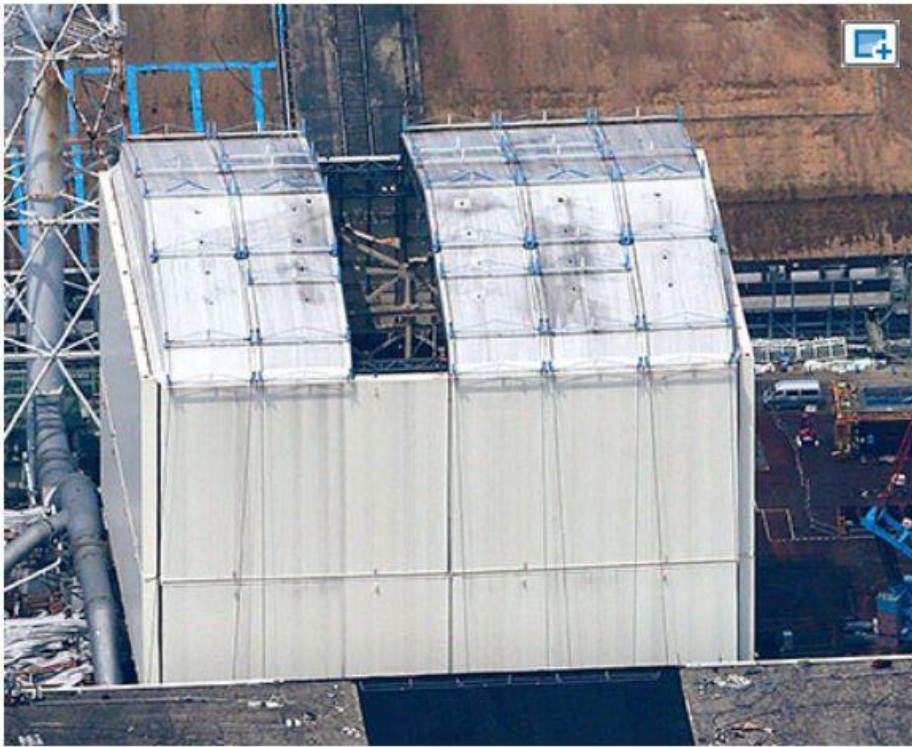
The interior of the No. 1 reactor building of the Fukushima No. 1 nuclear power plant can be seen from above after a canopy panel was removed on July 28. (Eiji Hori)
