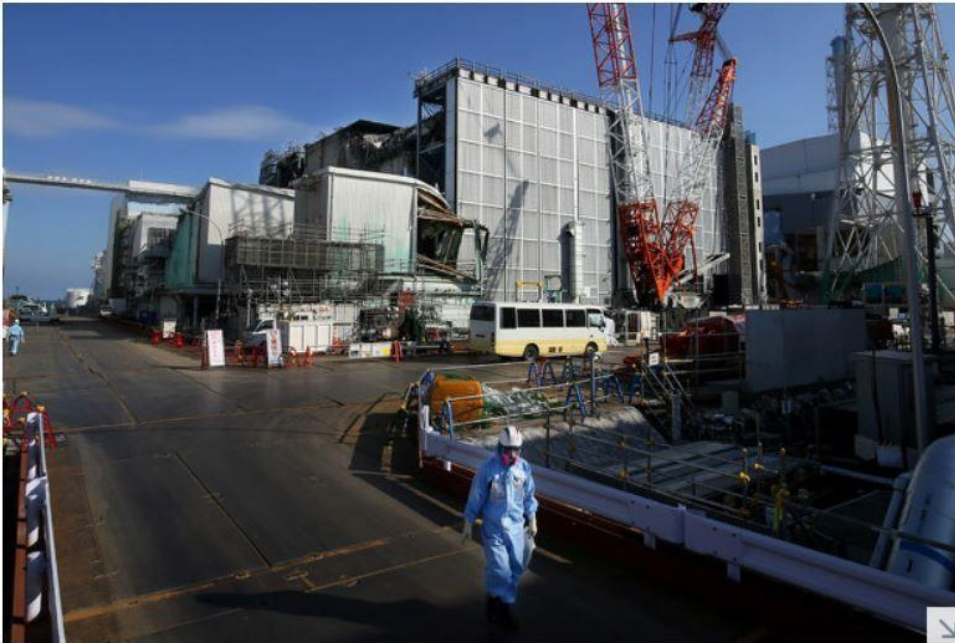
The No. 3 reactor building at the Fukushima No. 1 nuclear plant is seen on Feb. 23, 2016. (Mainichi)
