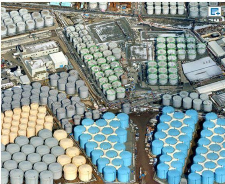
Rows of massive tanks storing radiation contaminated water line at the Fukushima No. 1 nuclear power plant in February. (Satoru Semba)
