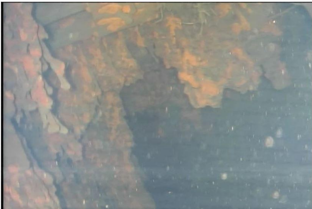
Material that appears to be nuclear fuel debris hangs like an icicle from the bottom of the pressure vessel of the No. 3 reactor at the Fukushima No. 1 nuclear power plant. (Provided by the International Research Institute for Nuclear Decommissioning)
