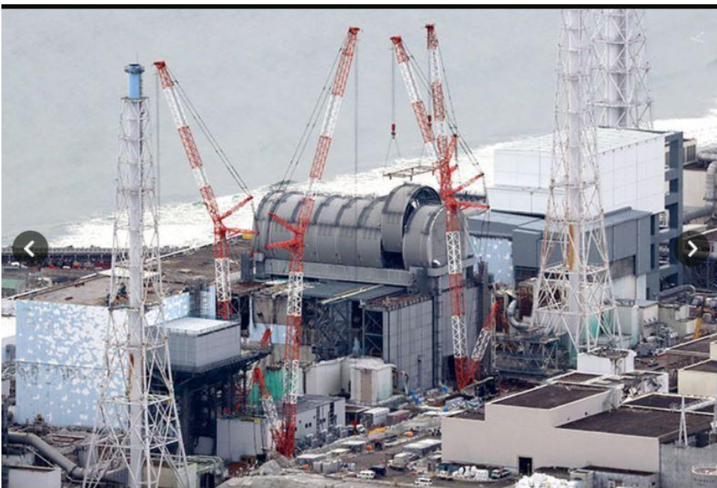
The final pieces of a jelly roll-shaped cover are being put in place atop the most damaged nuclear reactor, the No. 3 reactor of the Fukushima No. 1 nuclear power plant in Okuma, Fukushima Prefecture, on Jan. 25. (AP Photo)
