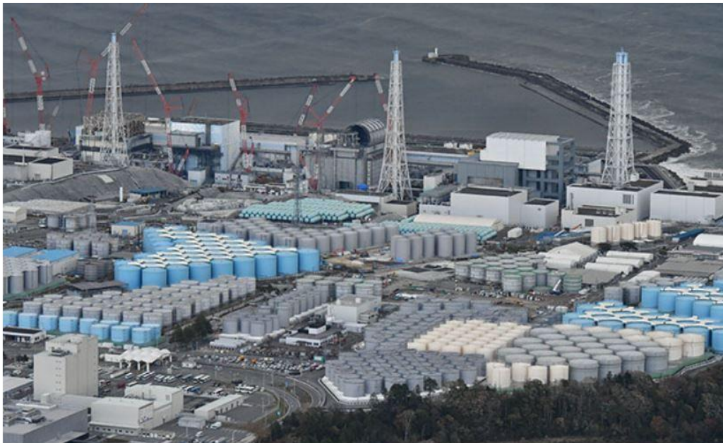
Rows of storage tanks on the grounds of the Fukushima No. 1 nuclear power plant contain water contaminated by radioactive materials. (Asahi Shimbun file photo)
