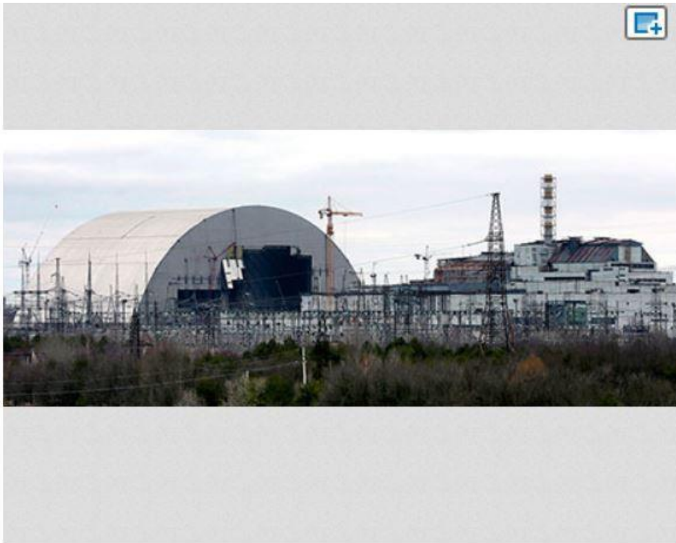
The semicylindrical shelter to the left will eventually cover the No. 4 reactor that is now encased in a concrete sarcophagus. (Yasuhiro Sugimoto)
