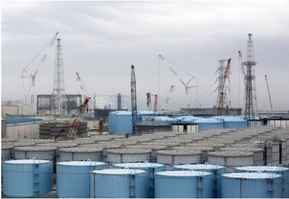
Storage tanks of contaminated water stand at Tepco's Fukushima No. 1 nuclear power plant. Tepco estimates that at the current rate it will run out of tank space in 2020, and a decision must be made on what to do with the water well before then. | BLOOMBERG
