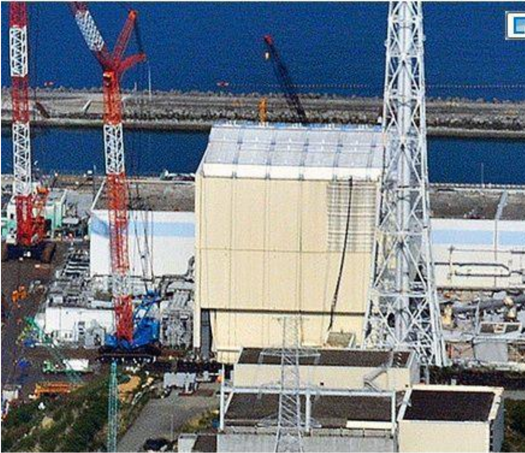
The cover over the No. 1 reactor building of the Fukushima No. 1 nuclear power plant in June 2014 (Asahi Shimbun file photo)
