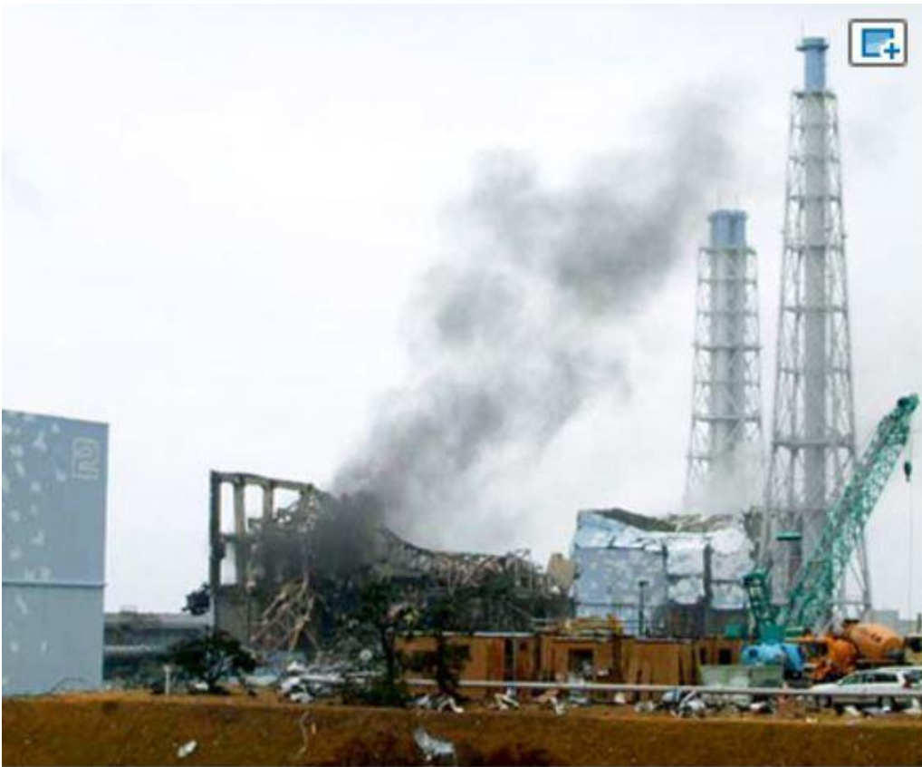
The No. 3 reactor at the Fukushima No. 1 nuclear power plant was damaged by an explosion in March 2011. (Provided by Tokyo Electric Power Co.)
