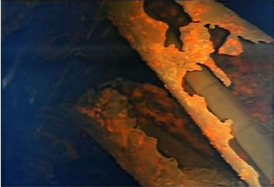
Severely damaged parts of a device once used to move control rods are stuck in a hole inside the pressure vessel of the No. 3 reactor at the Fukushima No. 1 nuclear plant. (Provided by International Research Institute for Nuclear Decommissioning)
