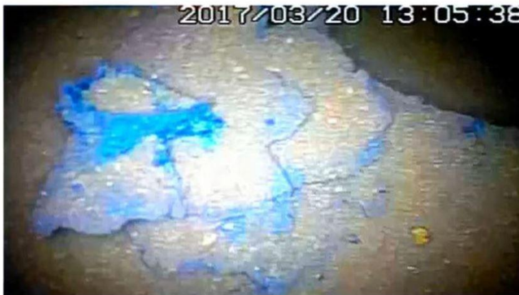
What appears to be sand has piled up on a pipe at the bottom of the containment vessel of the No. 1 reactor at the Fukushima No. 1 nuclear power plant. This image was taken by a survey robot on March 20. (Provided by the International Research Institute for Nuclear Decommissioning)
