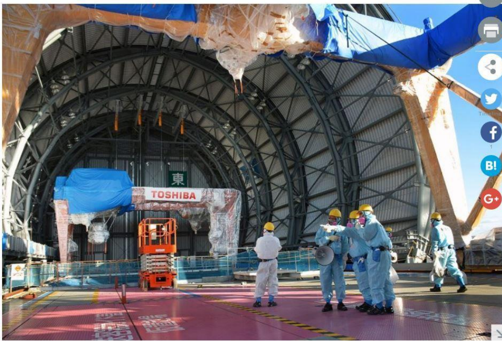
Fuel removal equipment is seen beneath a semi-cylindrical cover atop the No. 3 reactor building. (Mainichi)
