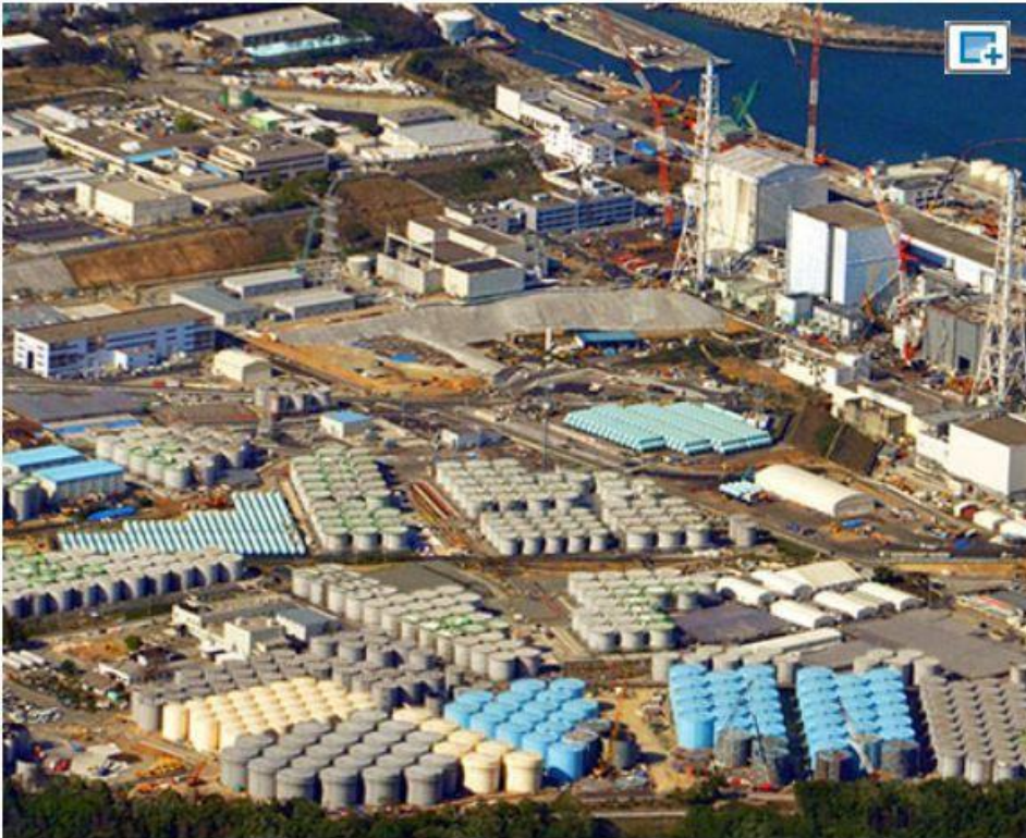
Rows of tanks holding contaminated water at the Fukushima No. 1 nuclear power plant (Asahi Shimbun file photo)
