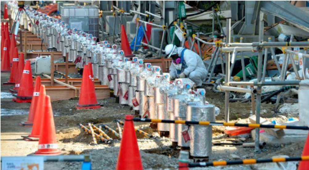
Devices to freeze the earth are set up on the southern side of the No. 4 reactor building at Tokyo Electric Power Co.'s Fukushima No. 1 nuclear power plant in Fukushima Prefecture in 2014. (Pool)
