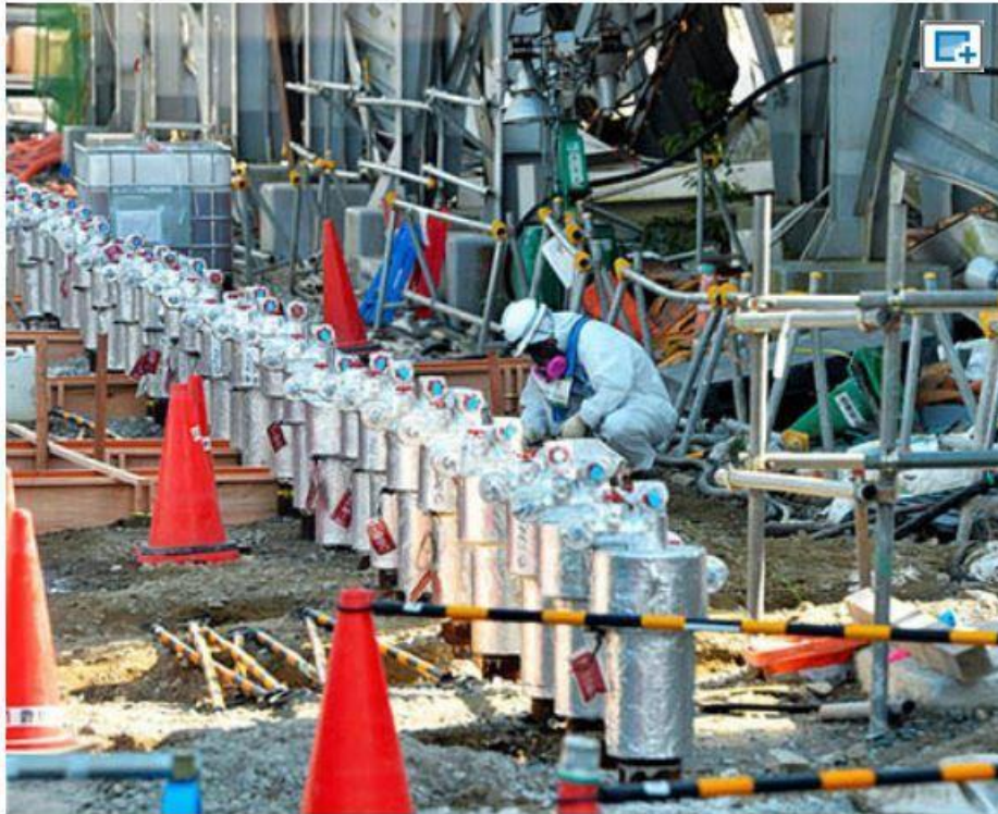
Pipes installed south of the No. 4 reactor building to create an underground frozen soil wall at the Fukushima No. 1 nuclear power plant (Pool)
