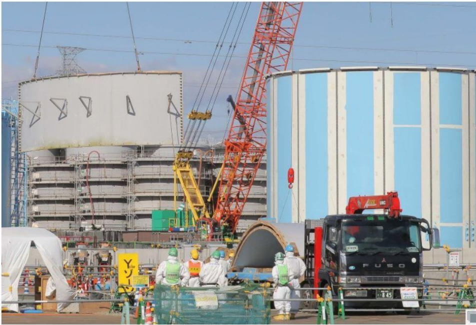
Workers bring in a new water tank, right, as a replacement for an old contaminated water tank at TEPCO's No. 1 nuclear power plant in the town of Okuma in Fukushima Prefecture on Feb. 24, 2017. (Mainichi)
