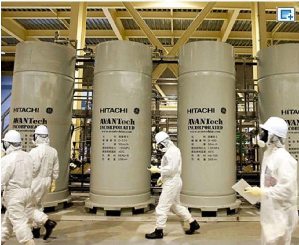
Equipment to decontaminate radioactive groundwater collected from subdrains set up around the main buildings of the Fukushima No. 1 nuclear power plant in Okuma, Fukushima Prefecture, last October. (Asahi Shimbun file photo)
