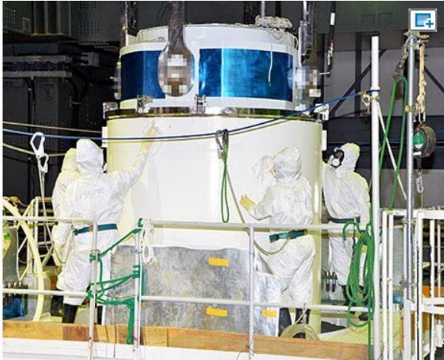
Workers wipe water from a cask containing nuclear fuel that was removed from the No. 4 reactor at the Fukushima No. 1 nuclear power plant on Dec. 20. (Pool)
