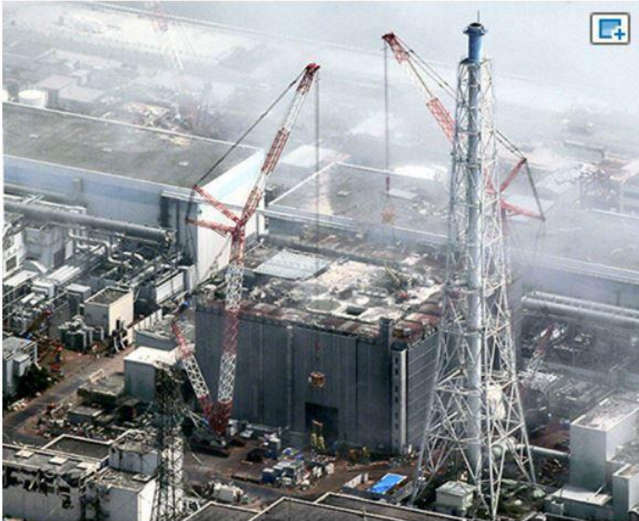
Two cranes are used to remove a huge piece of debris from the nuclear fuel storage pool of the No. 3 reactor building at the Fukushima No. 1 nuclear power plant on Aug. 2. (Tatsuya Shimada)
