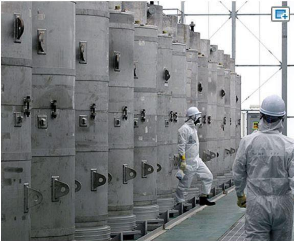
Equipment to remove radioactive substances from contaminated water stored at the Fukushima No. 1 nuclear power plant (Pool)
