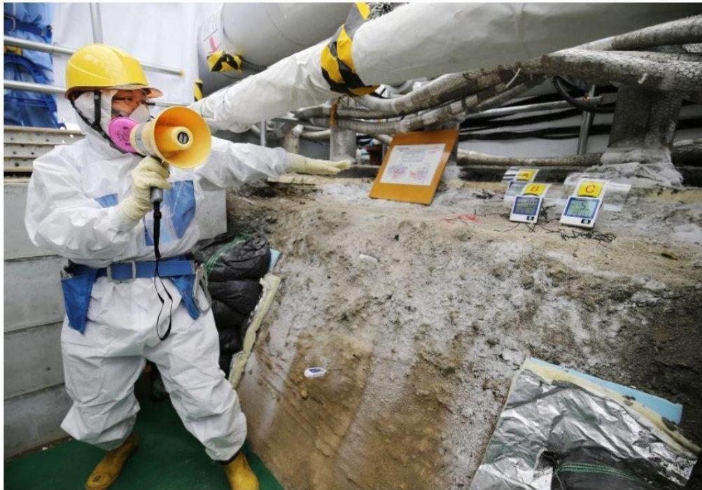
A Natural Resources and Energy Agency official explains the state of the ice wall meant to surround the reactor buildings at the Fukushima No. 1 Nuclear Power Plant, on Nov. 21, 2016. (Pool photo)
