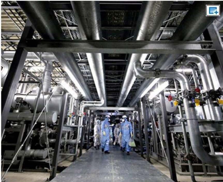
A large number of pipes and freezing equipment take up much of the space of Tokyo Electric Power Co.'s refrigerator plant at the embattled Fukushima No. 1 nuclear power plant on Feb. 19. (Yasuhiro Sugimoto)
