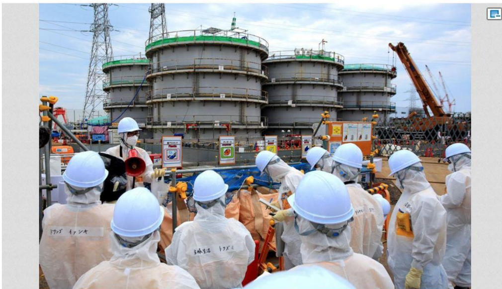
Reporters observe the dismantling of bolted flange-type tanks to store radiation-contaminated water at the Fukushima No. 1 nuclear power plant during a media tour Sept. 4. (Pool)
