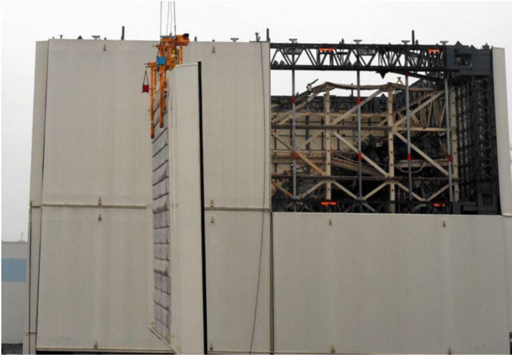
The outer layer of the crippled No. 1 reactor building at the Fukushima No. 1 nuclear power plant is exposed as Tokyo Electric Power Co. removes one of the panels covering the facility at 6:22 a.m. on Sept. 13. (Pool)
