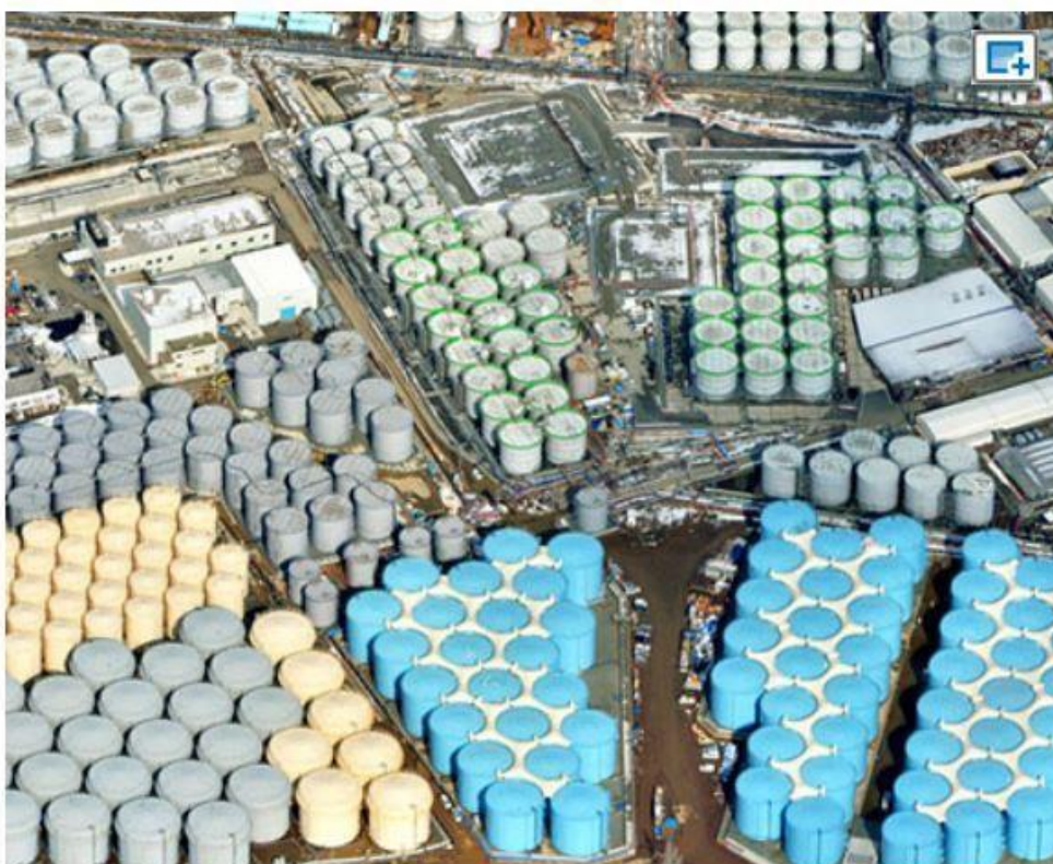
Rows of massive tanks storing radiation contaminated water line the compound of the Fukushima No. 1 nuclear power plant in early February. (Satoru Semba)
