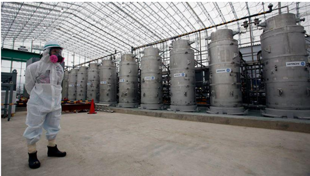
A Tokyo Electric Power Co. official wearing radiation protection gear stands in front of Advanced Liquid Processing Systems during a press tour at the Fukushima No. 1 nuclear power plant in 2014. (AP file photo)
