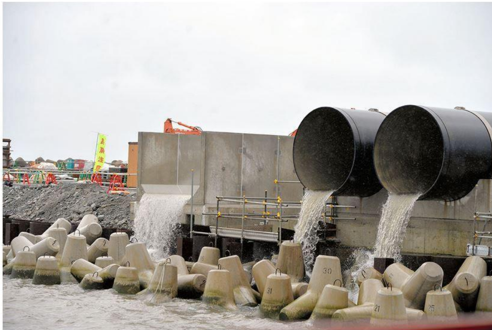
Rainwater is discharged from newly constructed drainage outlets into the plant's harbor during a media tour at the Fukushima No. 1 nuclear power plant on April 4. (Pool)
