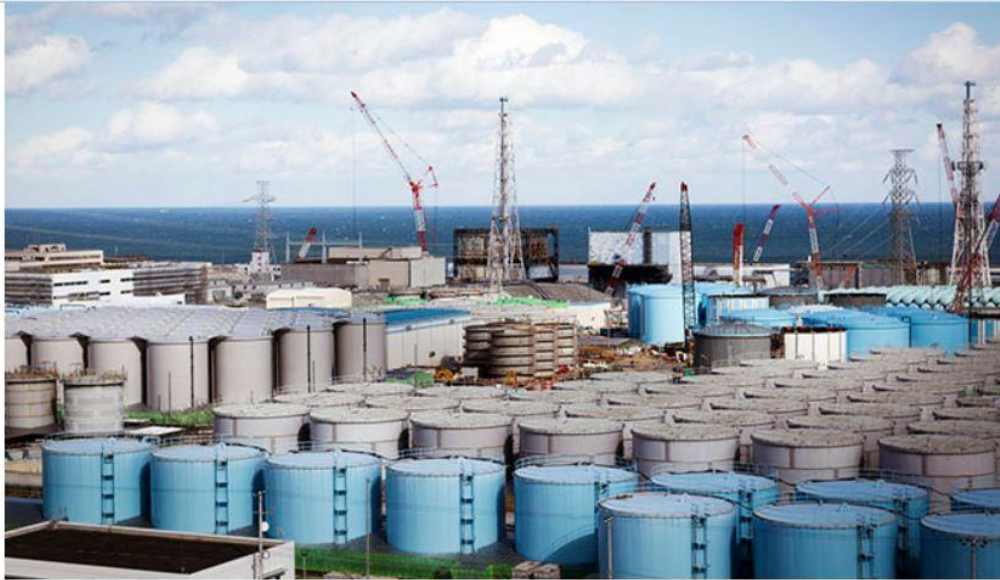
Tanks for storing contaminated water, with Reactors 1 and 2 in the background at the Fukushima Daiichi Nuclear Power Station in Fukushima, Japan, Feb. 21, 2017. Japanese officials wrestle with what to do with the ever-growing pile of radioactive waste at the nuclear power station, six years after the accident there. (Ko Sasaki/ © 2017 The New York Times)
