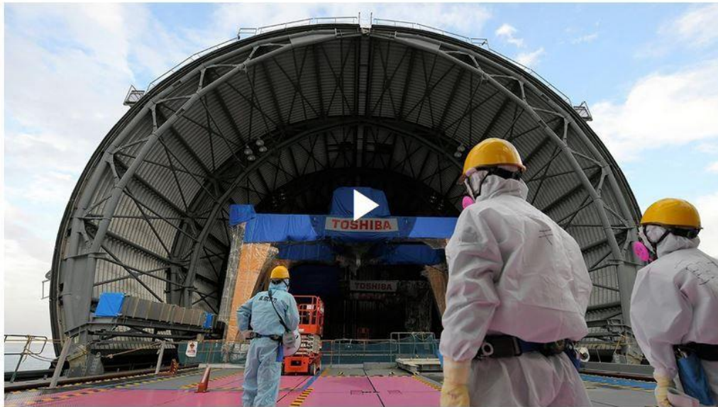
Media representatives walk on top of the No. 3 reactor building at the Fukushima No. 1 nuclear power plant where a huge dome is being constructed over the storage pool for spent nuclear fuel. (Video footage by Shigetaka Kodama)
