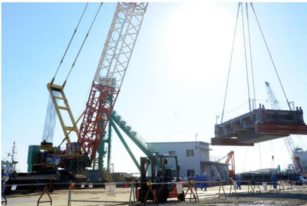
Steel frames are transported at the Fukushima No. 1 nuclear power plant on Dec. 20 to prepare for work to retrieve spent nuclear fuel from the storage pool of the damaged No. 3 reactor building. (Pool)
