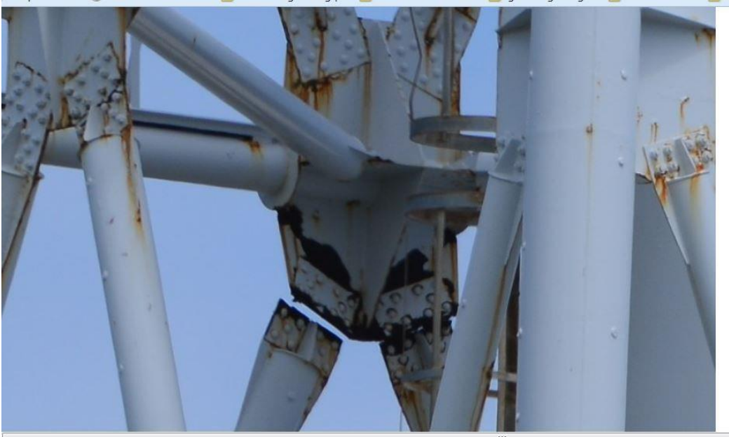
The fractured steel beam section of the exhaust stack pillar at the No. 1 and 2 reactors of the Fukushima No. 1 Nuclear Power Plant. (Photo courtesy of TEPCO)
