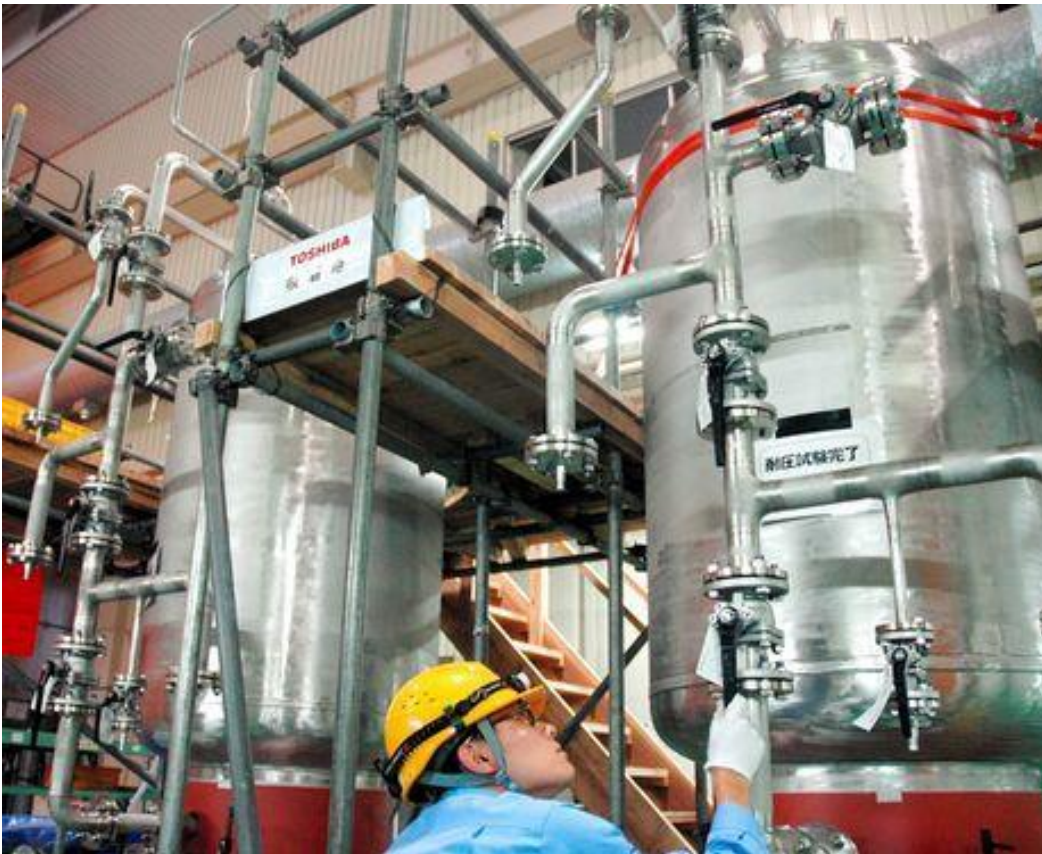
Part of the multinuclide removal equipment to be installed at the Fukushima No. 1 nuclear plant. (Asahi Shimbun file photo)
