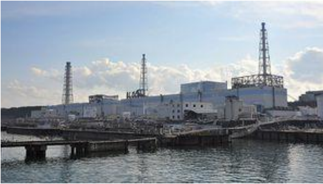
Damaged Tokyo Electric Power Co (TEPCO) number 1 daiichi nuclear power plant at Okuma town in Fukushima prefecture (AFP Photo)
