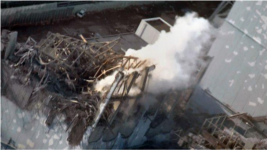
The damage to TEPCO's No.1 Fukushima nuclear power plant's third reactor building in the town of Okuma, Fubata district in Fukushima prefecture (AFP Photo)
