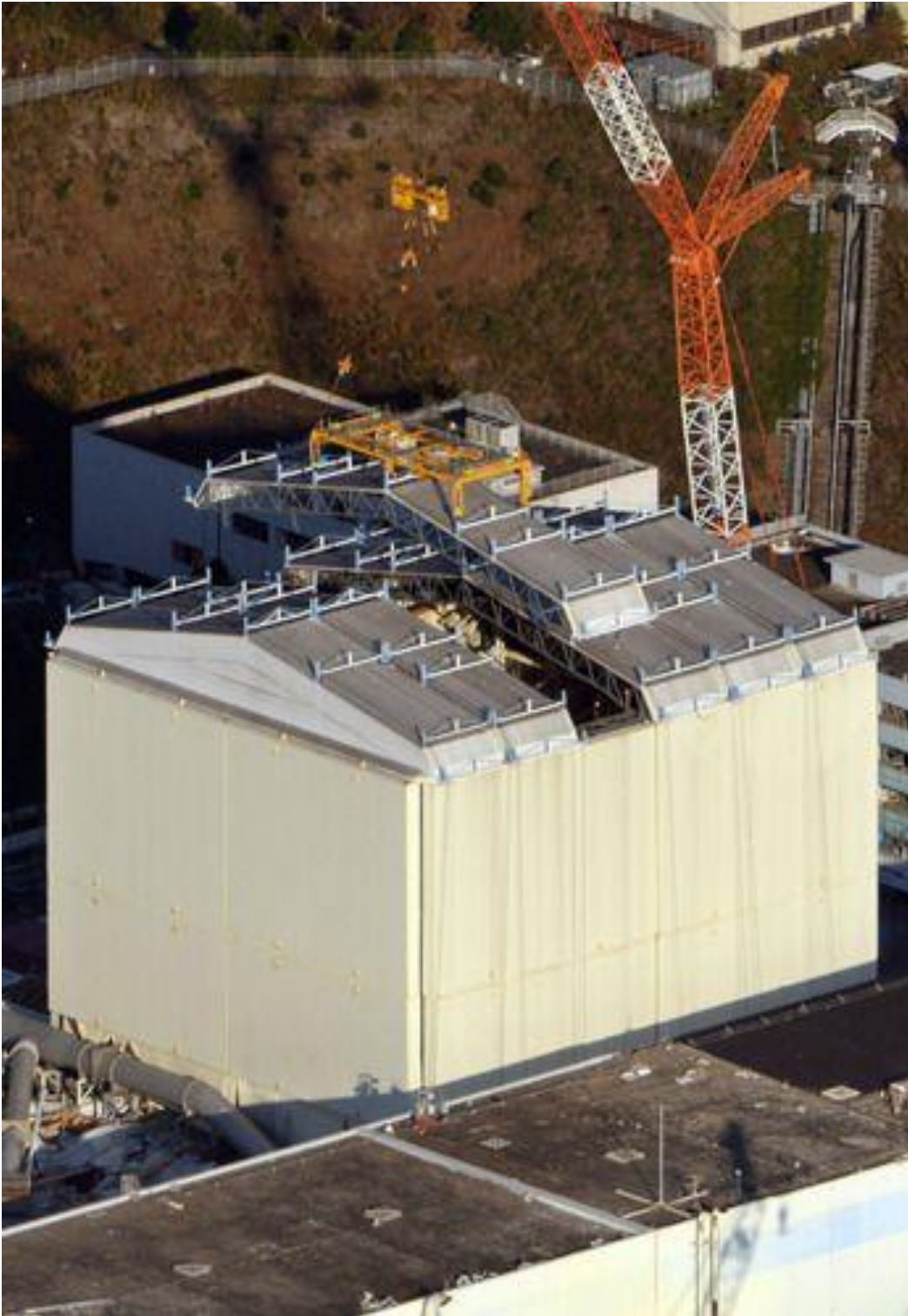
Part of the cover over No. 1 reactor of Fukushima No. 1 Nuclear Power Plant is removed, revealing massive debris inside the reactor on Oct. 31. (Mainichi)
