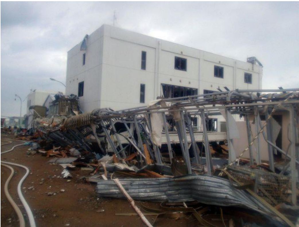
A destroyed building of TEPCO's Fukushima Daiichi (No. 1) atomic power plant at Okuma town in Fukushima prefecture (AFP Photo)
