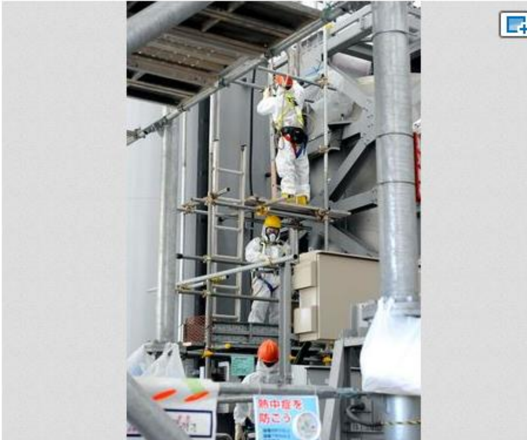
Workers inspect an ALPS device at the Fukushima No. 1 nuclear power plant. (Asahi Shimbun file photo)
