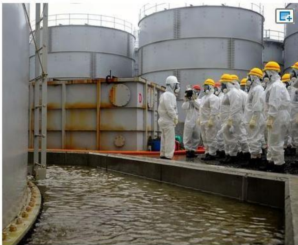
Storage tanks for contaminated water at the Fukushima No. 1 nuclear power plant. A barrier surrounding the tank is seen. (Pool)
