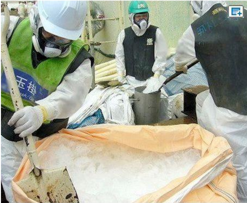
Workers prepare to pour ice into a trench filled with contaminated water in an attempt to create a sealant at the Fukushima No. 1 nuclear power plant in July. (Provided by Tokyo Electric Power Co.)
