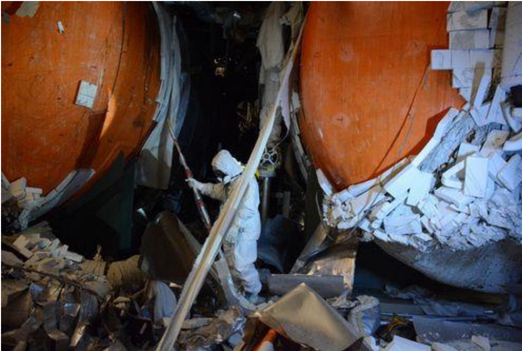
NRA officials inspect the fourth floor of the damaged No. 1 reactor building at the Fukushima No. 1 Nuclear Power Plant on May 31. (Photo courtesy of the NRA)
