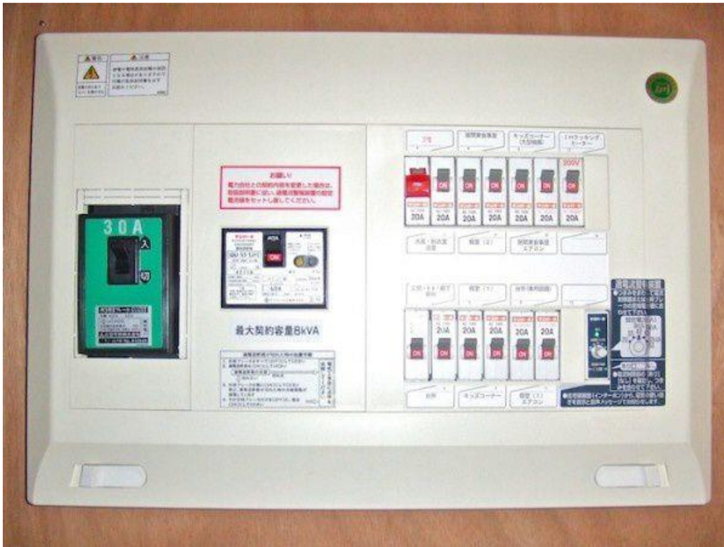
Power trip: electrical panel with 30-ampere main breaker switch
