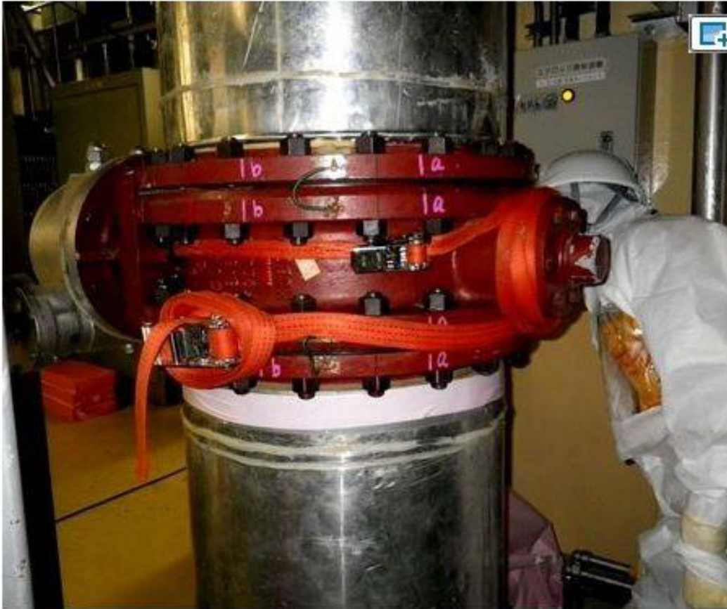
Fukushima prefectural government officials inspect the piping in the No. 5 reactor building at the Fukushima No. 1 nuclear power plant on July 7. (Provided by the Fukushima prefectural government)
