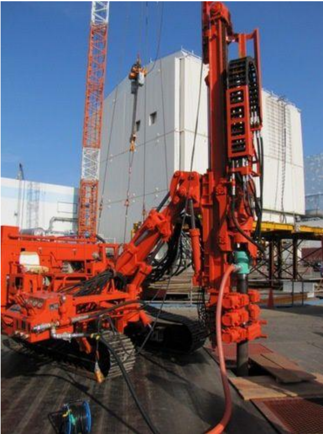
A heavy machine is used to drill a hole on June 2 near the No. 1 nuclear reactor building in which a frozen pipe is to be inserted to build an underground frozen wall at the Fukushima No. 1 Nuclear Power Plant. (Photo courtesy of Tokyo Electric Power Co.)
