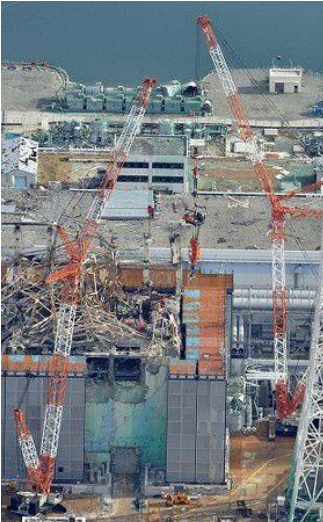
A crane (right) lifts a steel beam out of the Fukushima No. 1 nuclear plant's No. 3 reactor spent fuel pool on Dec. 20. (Mainichi)
