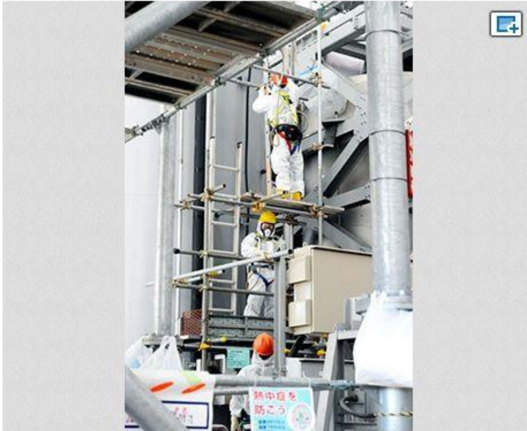
Workers clad in protective suits check the ALPS equipment at the Fukushima No. 1 nuclear power plant in November 2013. (Asahi Shimbun file photo)
