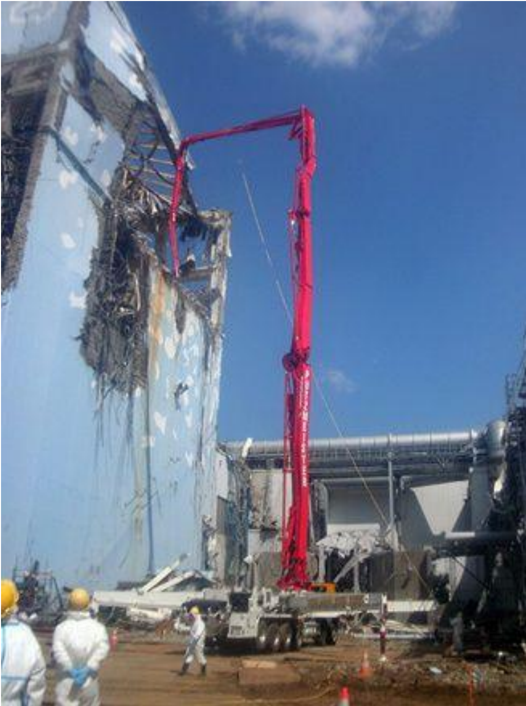
Workers using a German-made pump to pump water from the spent fuel pool in Unit 4 at Fukushima No.1 (Dai-Ichi) nuclear power plant in the town of Okuma in Fukushima prefecture (AFP Photo)
