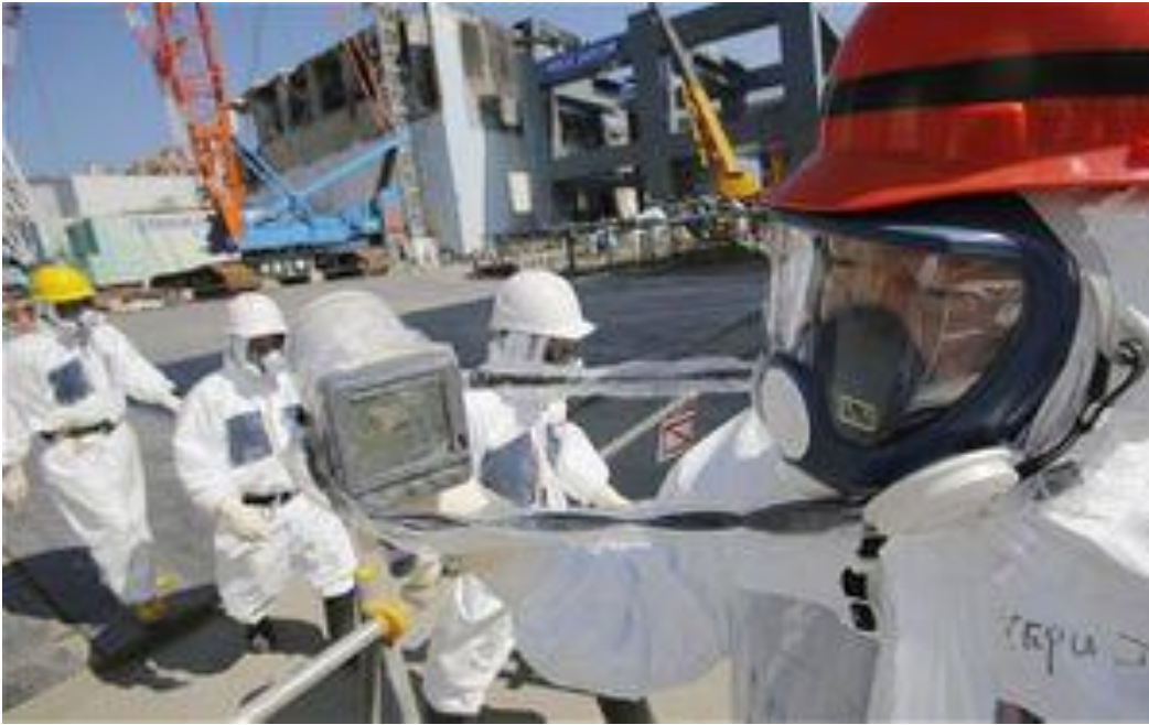
A radiation monitor indicates 114.00 microsieverts per hour near No.4 reactor and it's foundation construction Photo: Reuters By Julian Ryall, Fukushima Nuclear Plant, Japan
