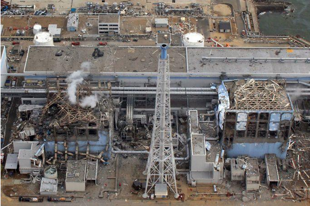
The stricken Tokyo Electric Power Company (TEPCO) Fukushima daiichi No.1 nuclear power plant reactor number three (L) and four (R), with smoke rising from number three at Okuma town in Fukushima prefecture (AFP Photo)
