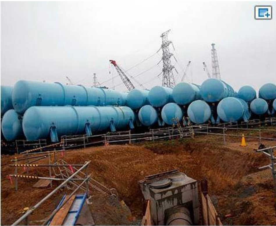
Tanks storing contaminated water are seen at the Fukushima No. 1 nuclear power plant in Fukushima Prefecture on Nov. 12. (AP Photo/ Pool)
