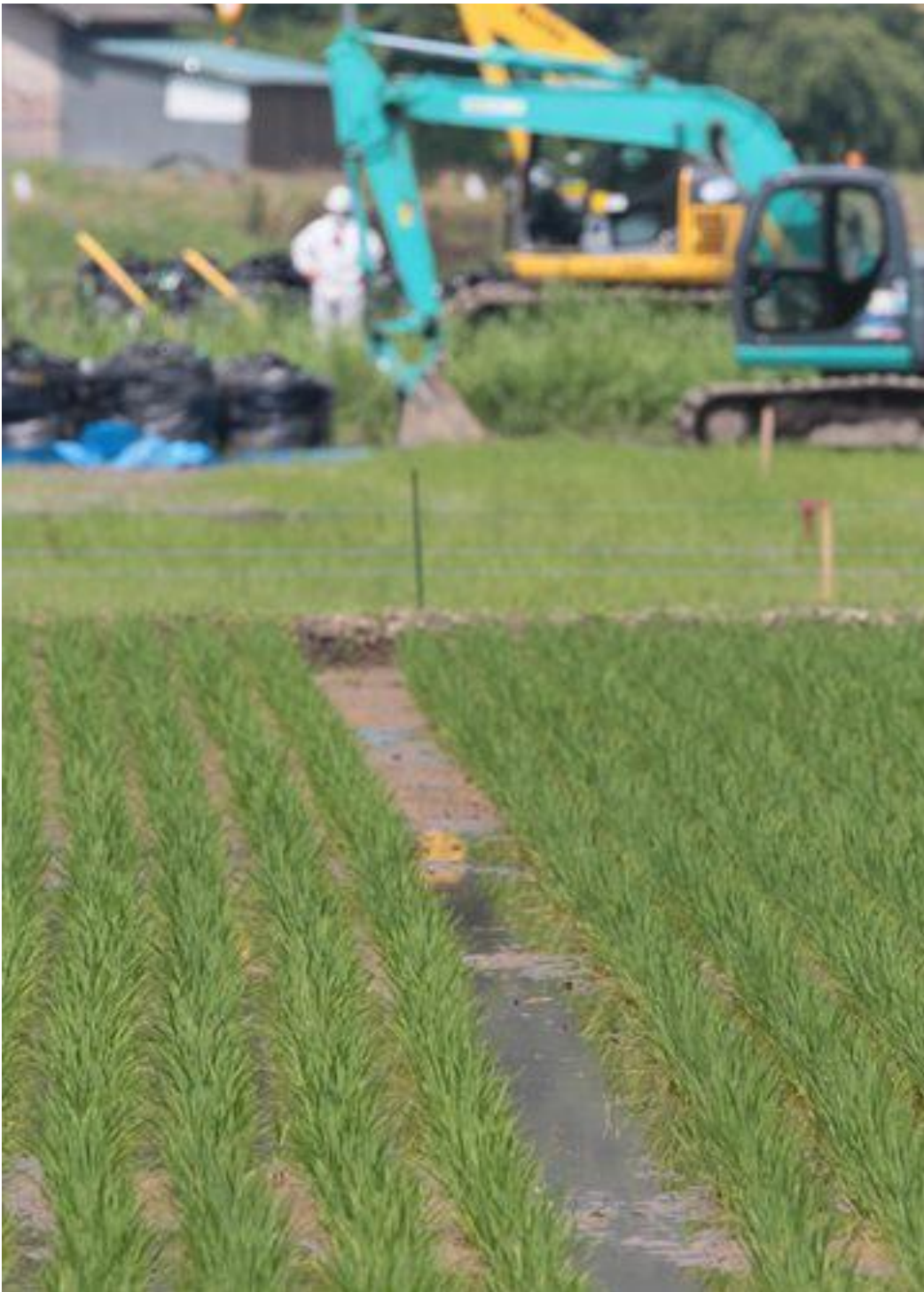
Rice plants are seen at a testing paddy in Iitate, Fukushima Prefecture, in this July 28 file photo, as decontamination work progresses in the area. (Mainichi)
