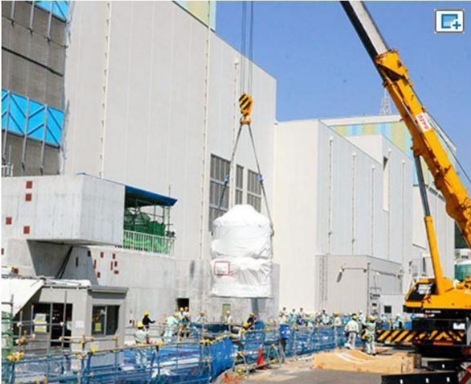
An iodine filter to reduce the release of radioactive materials in event of an accident is installed at the Shimane nuclear power plant in Matsue, Shimane Prefecture, on April 27. (Ryo Isshiki)
