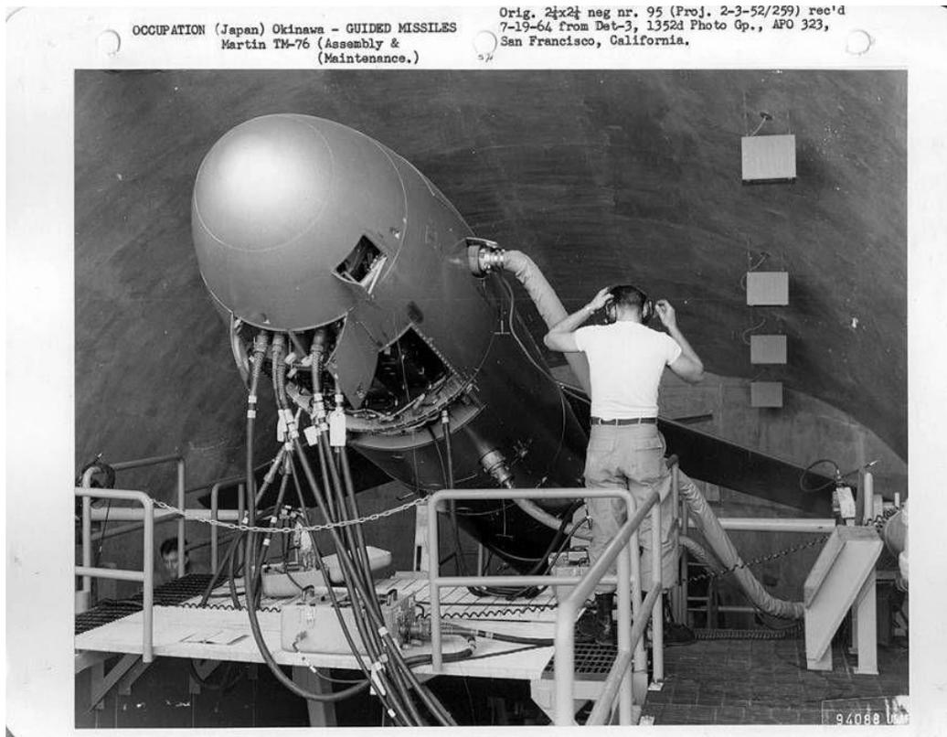
Technicians work on a Mace B cruise missile on Okinawa in April 1962. Carrying a 1-megaton W28 nuclear warhead, the rocket-boosted, jet-propelled Mace missile could be fired at six minutes' notice. | NARA, STILL PICTURES UNIT, RECORD GROUP 342B, BOX 1470
